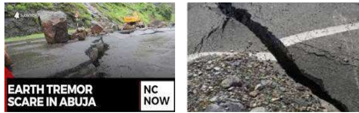
Plate I: Aftermath of the Earth Tremor in Part of Federal Capital Territory Abuja, Nigeria in the year 2018 (Daily Trust, newspapers, 2018)
