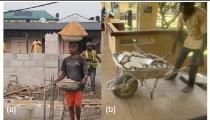
Figure 1: Transportation of site construction materials using (a) head pan and (b) wheelbarrow
