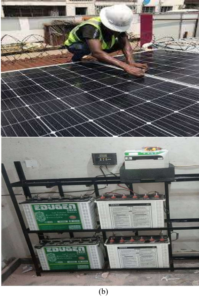
Figure 1 Experimental Setup and PV System Layout (a) The experimental setup used for data measurement (b) Layout of a PV power system showing the separation and organization of cables from the PV module, and the integrated setup of the inverter and battery bank for power conversion, storage, and distribution.
